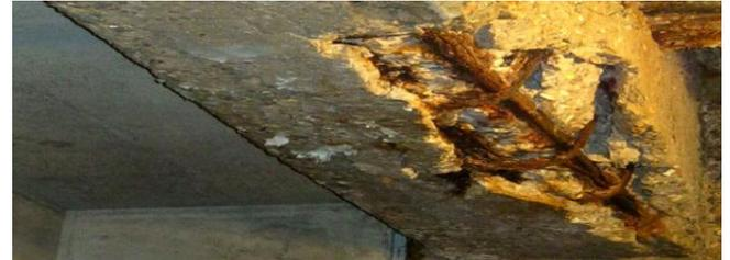
Fig -1: corroded steel embedded in concrete
