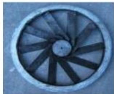
Figure 6: The schematic of the swirl plate in liquid column tower
