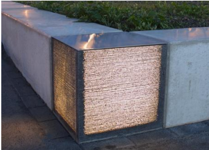
Figure 1: Piece of Transparent Concrete used in Fencing Wall.
