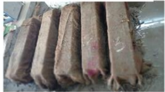
Fig 2: Curing of Concrete
