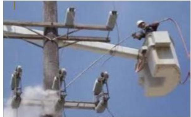
Fig.2b Dry Cleaning of insulator [10]
