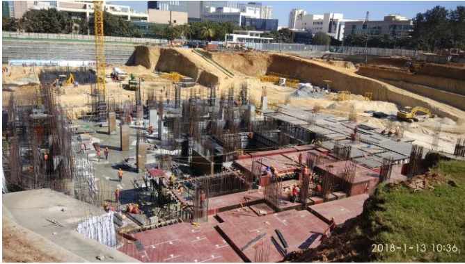
Fig -4: Table mould arrangement at site.
