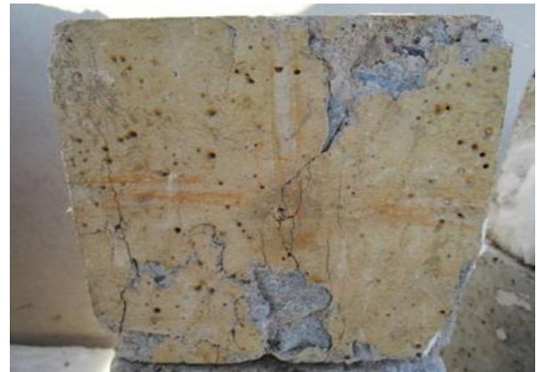
Figure 8.Sulfate corrosion for crumb rubber concrete
