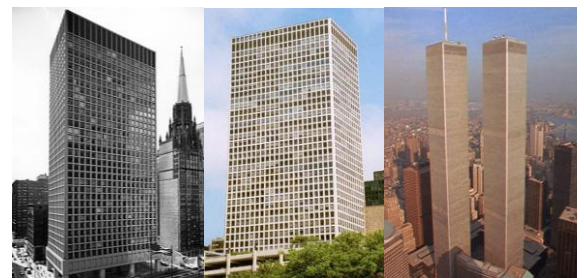
Fig -2: Framed Tube structure (a) Brunswick Building, Chicago (b) De Witt Chestnut Apartment, Chicago (c) World Trade Centre (1973-2001)
