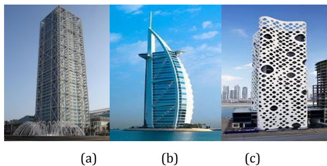
Fig -1: Exoskeleton structure (a) Hotel De Las Artes, Spain (b) Hotel Burj Al Arab, Dubai (c) O-14 Business Bay, Dubai
