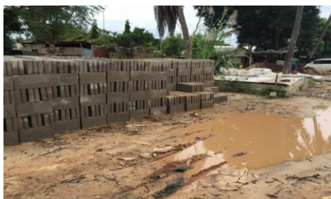
Figure - 1: Stacking of concrete blocks at Bunju area
