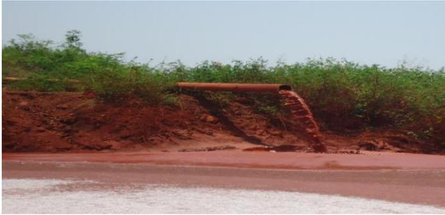
**Figure 2. Discharge of Red Mud as Slurry into the Pond**
