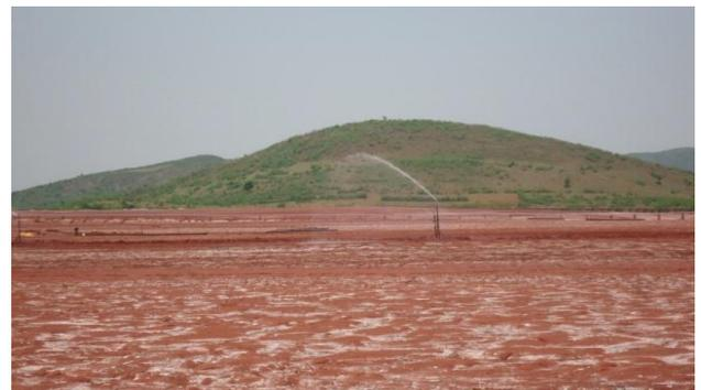
**Figure 4. Sprinkling system of red mud pond to prevent dust effect at Damanjodi**
