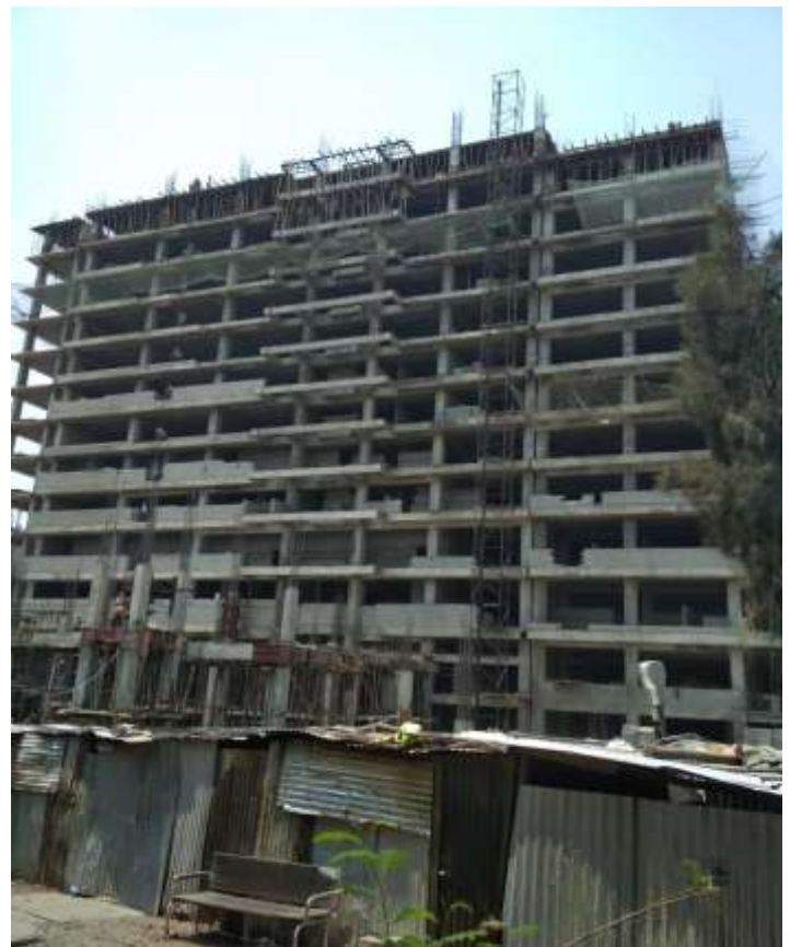
Figure 2: View of Gandhi Medical College Constructions Site.
