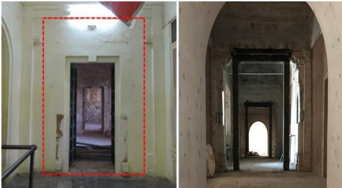
Fig -1: On Site Structural strengthening and circulation provision before and after.
