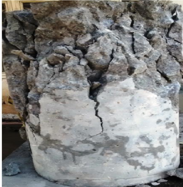
Figure 7. Failure pattern of traditional concrete
