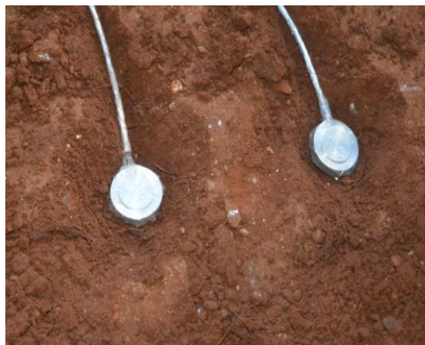
Fig - 2: Pressure cell installation
