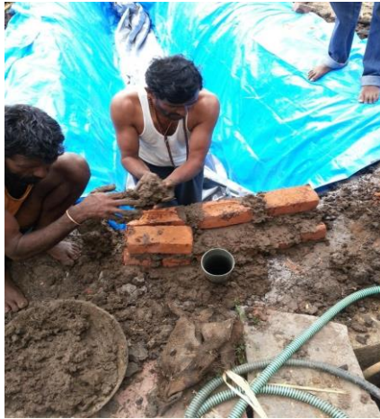
Fig -5 Installing inlet chamber
