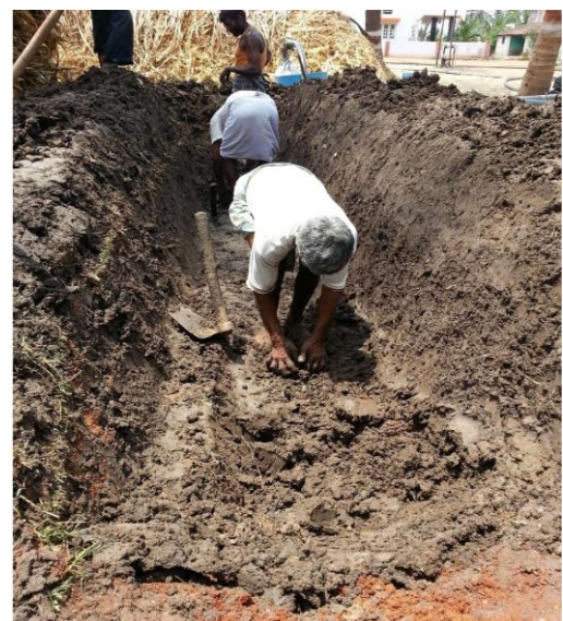
Fig -4 Digging of Bio Digester.
