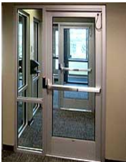
THREE ACCESS CONTROL MANTRAP SYSTEM
