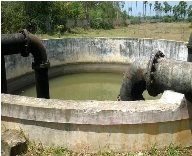
**Photograph 3.2.1: Raw water Collection sump at Treatment plant**
