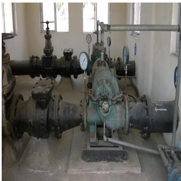
**Photograph 3.2.1: Raw water pumping by centrifugal pumps**
