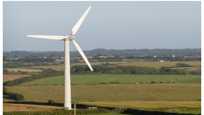
Figure -1: wind turbine
