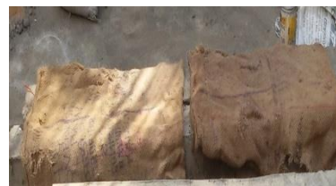
Fig 8:- Curing of beams
