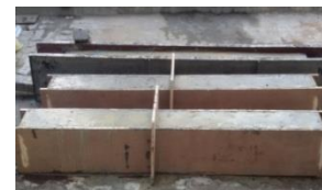
Fig 6:- Concrete surface is smoothed
