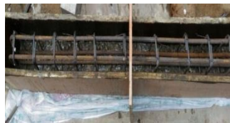
Fig 5:- Placing of reinforcement
