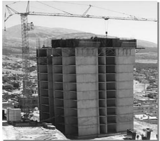
Fig-1: RC wall (Tunnel Form) Construction
