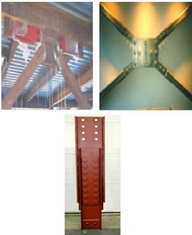
Fig -1: 1) Friction Dampers in Chevron Brace, 2) Friction Damper in Tension-Compression Brace, 3) Friction Damper for Tension-only Cross Brace
