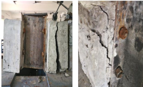
Fig.9 - Failure mode of bolt shaped shear connector
