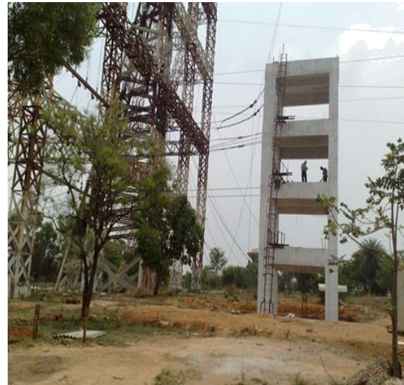
Figure1: Structure located at the tower testing facility CPRI Bangalore
