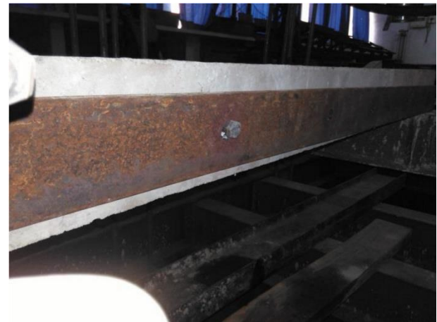
Fig. 7: Beam retrofitted with plates front and flipline plate.
