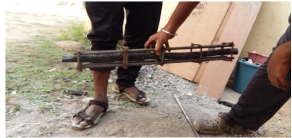
Figure 1: Placement of rubber tire tube inside reinforcement
