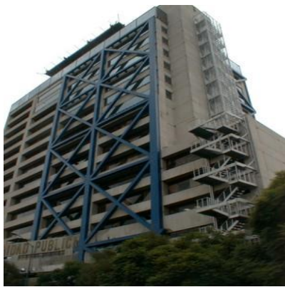
Figure 2 :- Centrally braced frame
