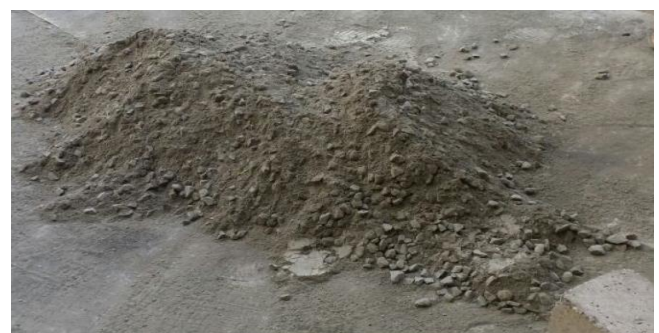
Fig-2: Mixing of concrete
