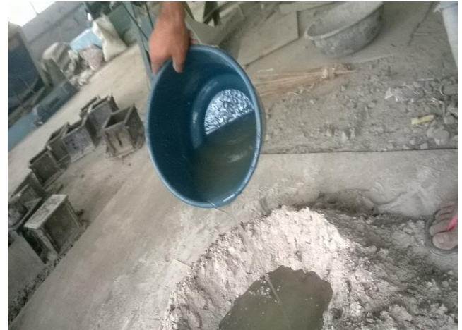
Fig.-4: Addition of Alkaline Solution
