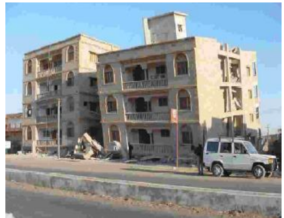
Fig -1: Damage to OGS building during Bhuj earthquake
