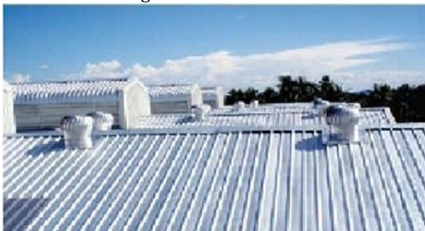
Fig.-7: Turbo Ventilator
