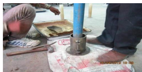
Fig.3 MODIFIED PROCTOR TEST
