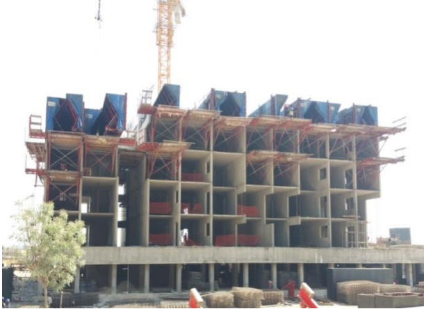
Figure 3 :- E1 Building During Tunnel Casting
