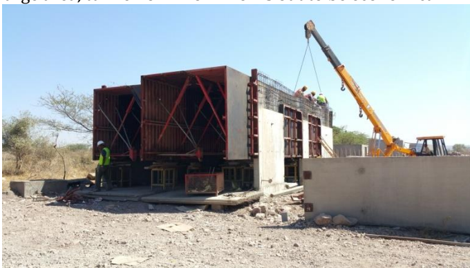
Figure 5 :- Transformer room using Tunnel Form
