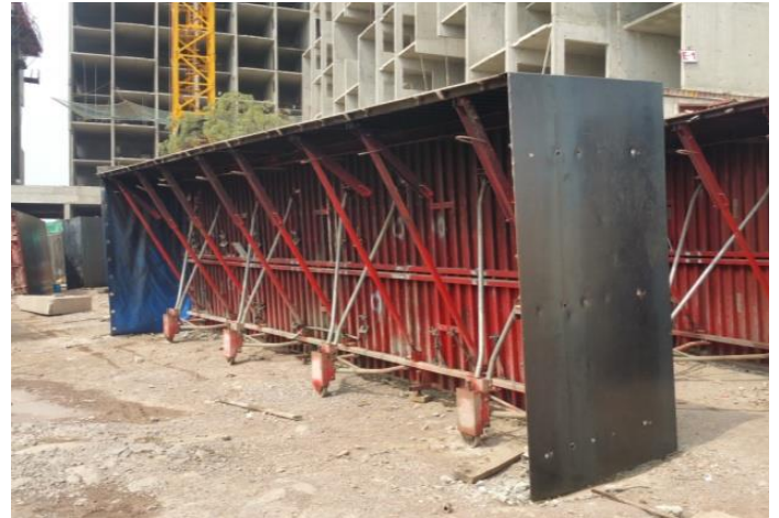
Figure 2 :- Tunnel Form at Site
