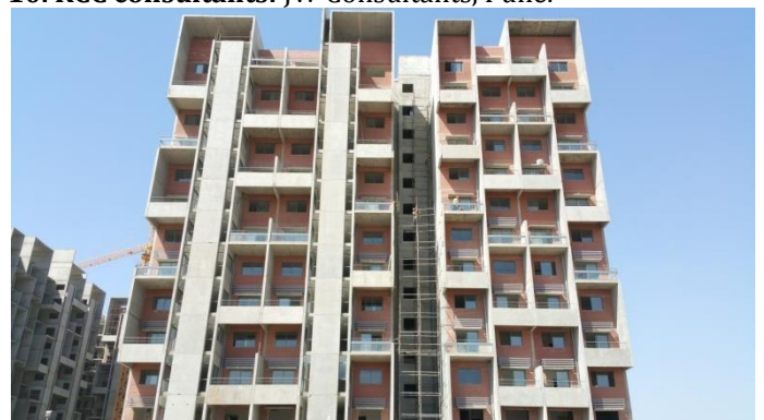
Figure 4 :- E1 Building in finishing stage
