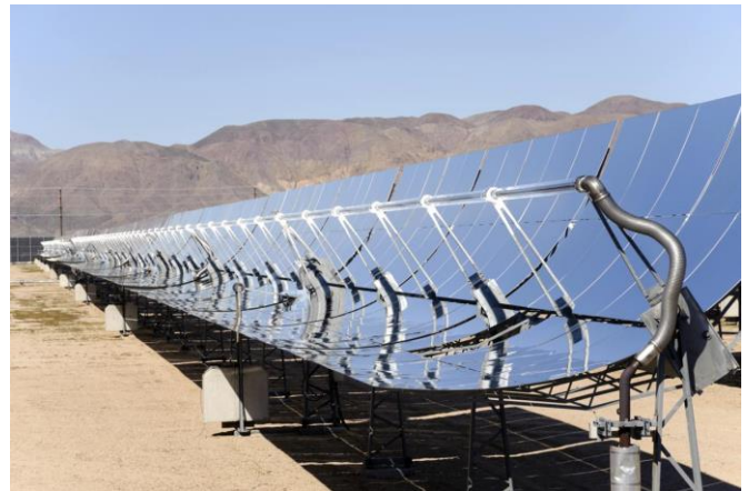
[Fig. 1 Parabolic trough concentrating solar collector]
