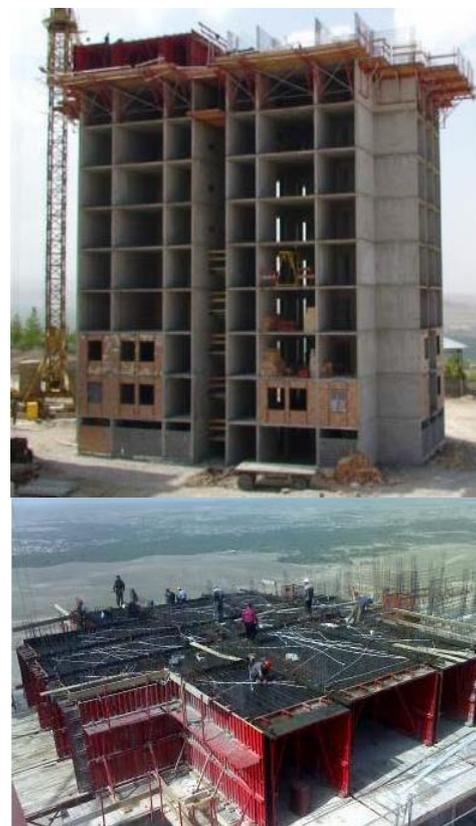
**Fig. 4 Tunnel form construction**
