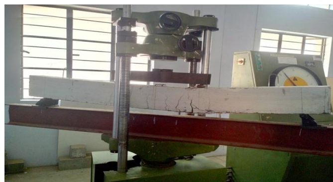
Fig -5: Crack Patterns Observed At Ultimate Load in Conventional Beam with Fiber at Soffit
