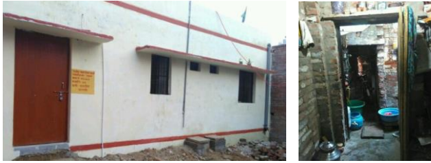
Figure 6: House constructed under RAY and transit accommodation of the beneficiary
