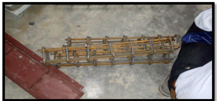
Fig 1 show reinforcement details of beams
