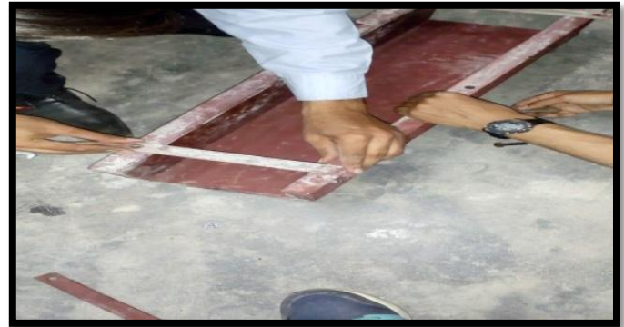
Fig.2 Preparing beam mould
