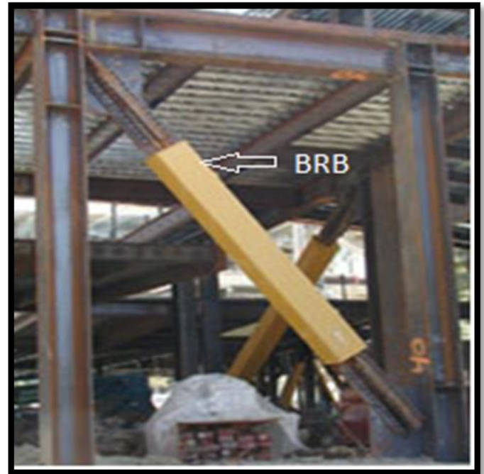
Figure 1. Buckling Restrained Bracing
