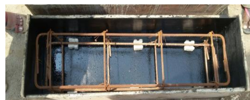
Figure 5 beam reinforcement and mould
