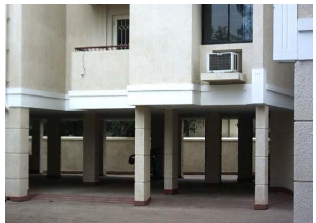
Fig-1.1 Typical Soft Storey in India
