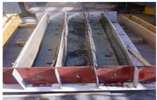
Figure-2. Mould for U-shape beam
