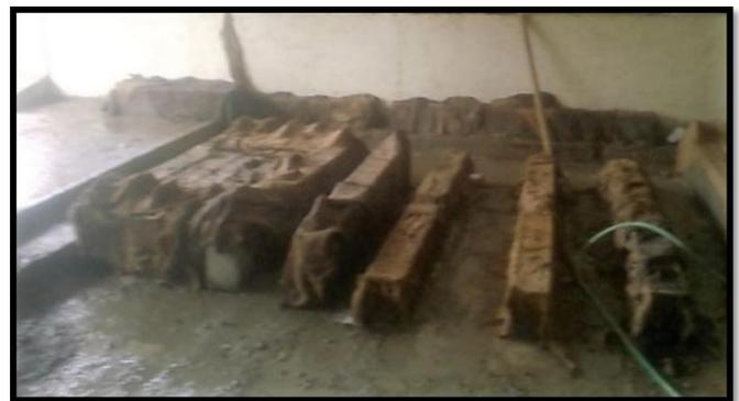
**Fig -4:** Curing of Beams
