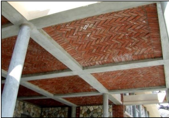
Fig-1: Typical view of Funicular Shell roof.
