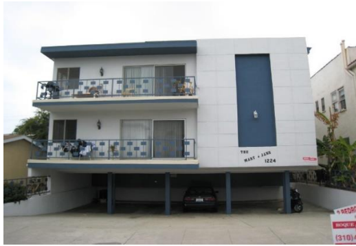
Fig.2: Example of Soft storey
