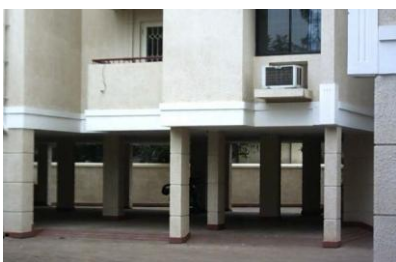
Fig -1: Photograph of stilt floor building.
