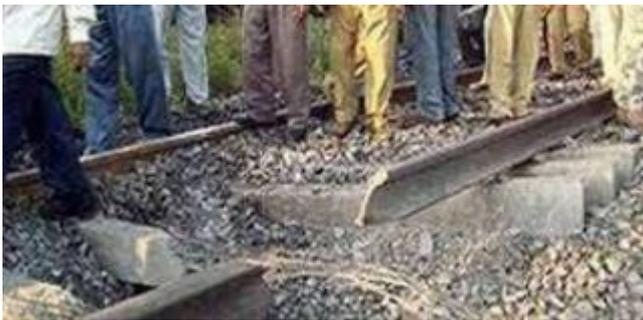
Fig -1: Crack in the railway track
