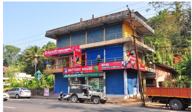
Fig- 1: Three storied building before collapse
