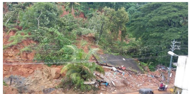
Fig- 2: Three storied building after collapse
