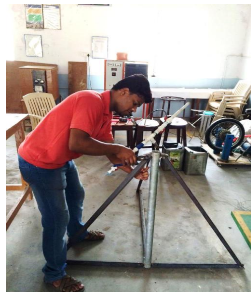
Fig.2. Base Frame installation
