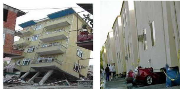
Figure: 2 Failure of soft storey
