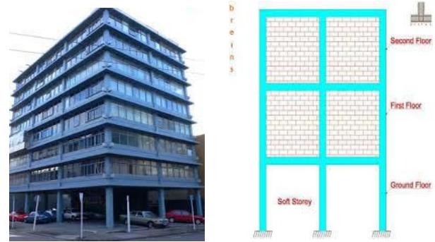
Figure: 1 Soft story buildings
