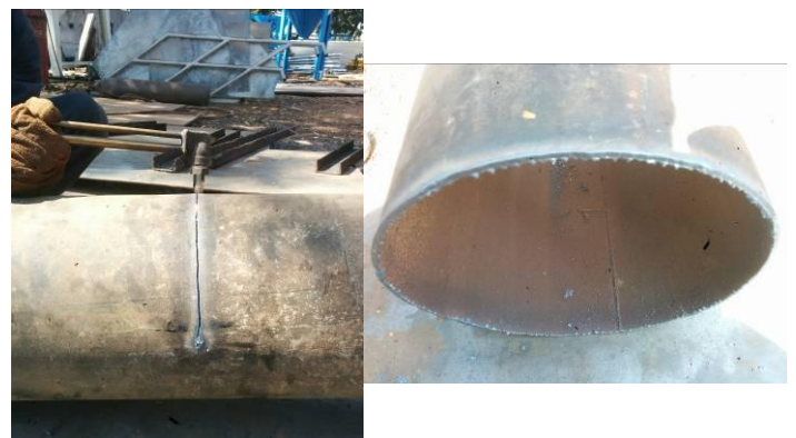
Figure C- View of pipe during and post cutting
